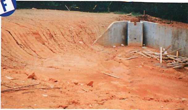
No vegetation. Perforated standpipe with gravel filter is missing.
