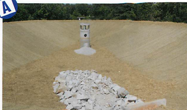
Perforated standpipe with gravel filter in place.
