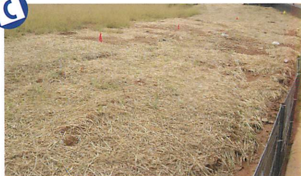
Good coverage of mulch and temporary grass, but runoff has exposed some areas.
