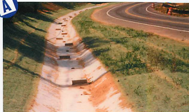
Excellent coverage with synthetic mats and vegetation.
