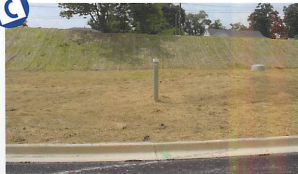
Matting applied to slopes, some areas exposed. Vegetation beginning, watering needed. Mulching in foreground pretty good.
