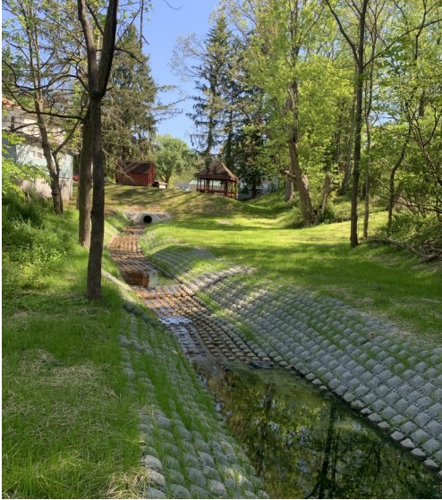
Drainage in the area of City Ave was upgraded to replace old and failing pipes with stabilized grass swales. Spring 2022
