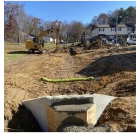
Concrete headwall installation during excavation of drainage swales in Maxwell Woods. Fall 2022
