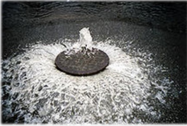
I&I adds too much water to a sanitary sewer system. This water sometimes comes out in sewer overflows, as shown here. Source: U.S. EPA, Boston, MA. "Eliminating Sanitary Sewer Overflows in New England."
