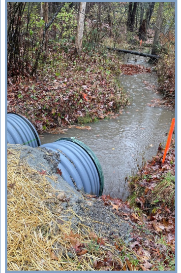
Post-Construction: Twin HP Dual Wall Pipes functioning as designed.
