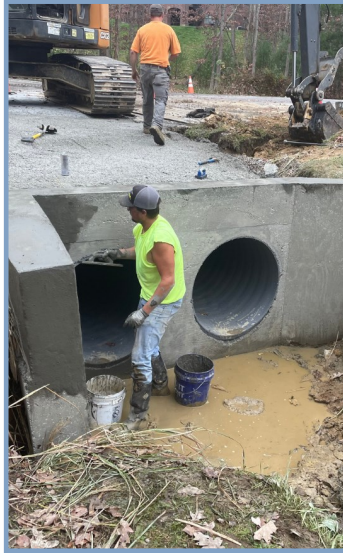
Construction: Installation of new headwall & HP Dual Wall pipe.
