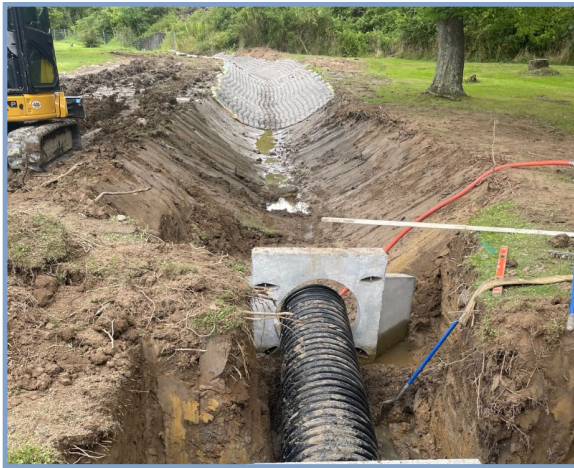
A new headwall and concrete matting being installed.
