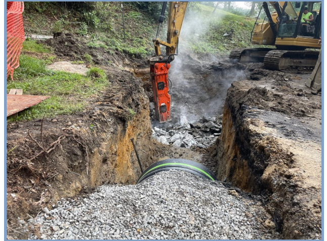
Crews preparing a ditch line for the new pipe installation.
