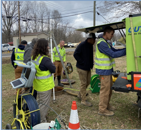
An environmental staff member operating the pipe inspection camera car to locate the break.
