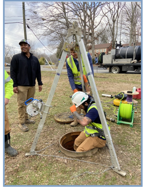
A repair team staff member entering a man-hole to assemble the pipe repair device.
